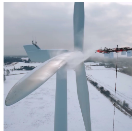
Figure: Drone de-icing of a wind turbine
