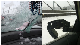
Figure: Ice falling from bridge cables
