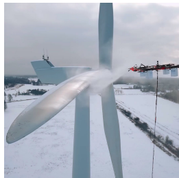
Figure: Drone de-icing of a wind turbine
